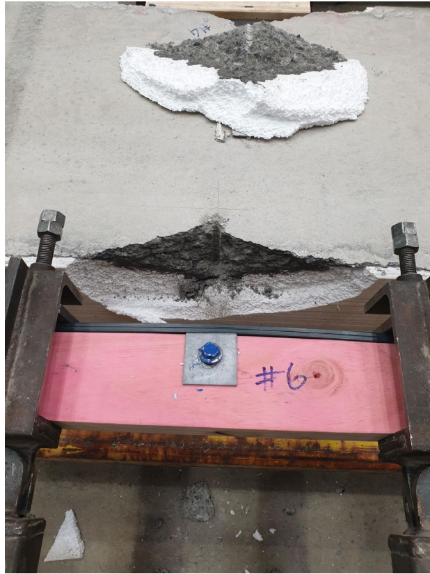
Figure 8. M10 x 140 mm Bowmac after failure in out-of-plane testing.
