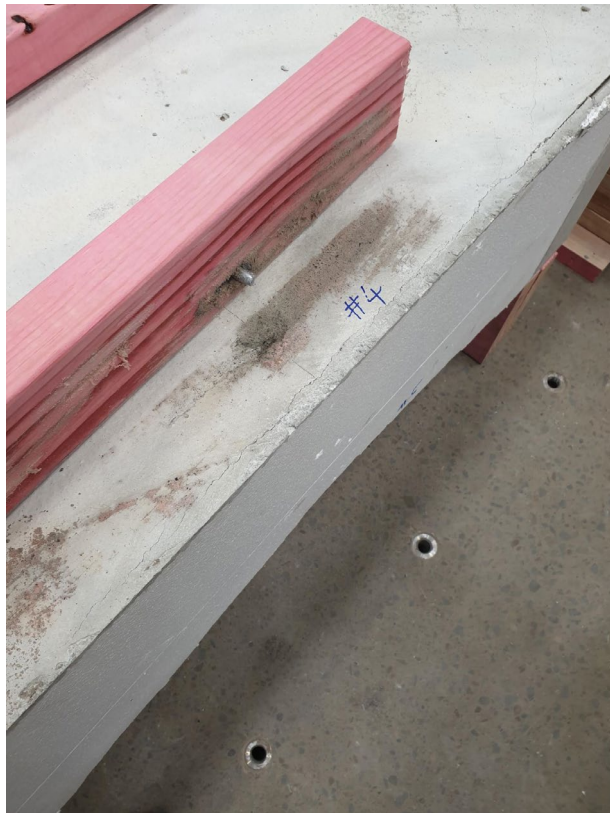
Figure 9. M10 X 140mm Bowmac after failure in-plane testing.
